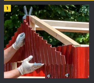
1 After marking the special pieces to cover the gable of the garden shed or tool shed, make the cuts without any problem, even if they are angled with respect to the inclination of the wave.
