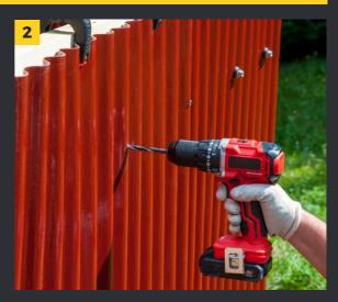
**5** Secure with hexagonal head screws and the special gaskets with washer and grommet that prevent rainwater from passing through. **4** With the sheet positioned on the frame underneath and held in place by clamps, insert the screws into the hole and tighten with a screwdriver. Calibrate the tightening so that the grommet is flush against the sheet without flattening the wave.
